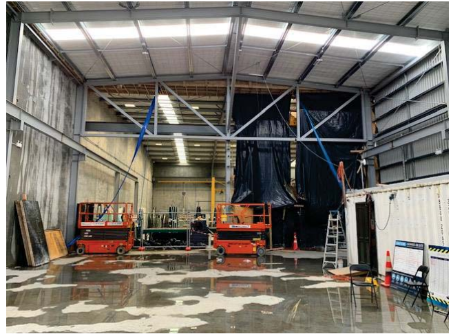
New - under construction
