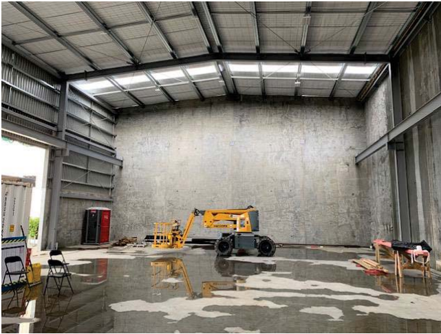
New - under construction
