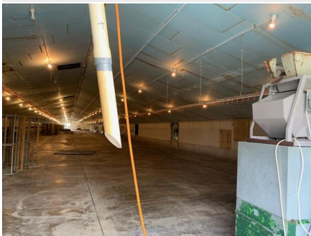
Internal - Original Shed
