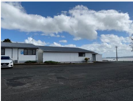
Office / Workshop External
