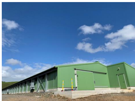
F Site Shed
