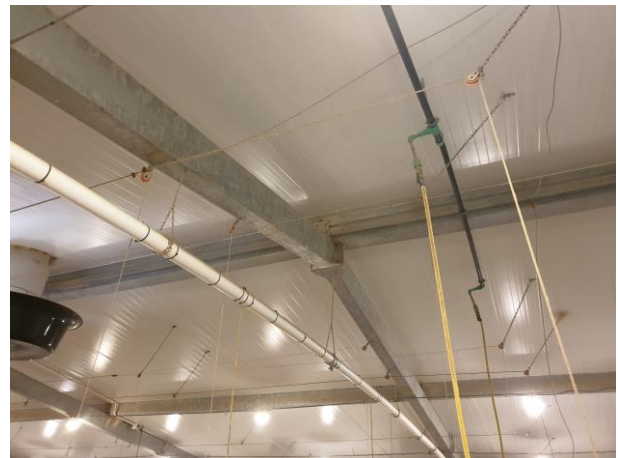
Typical interior construction
