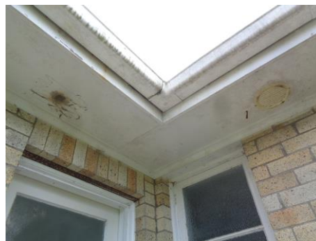
Grime to soffit and gutter
