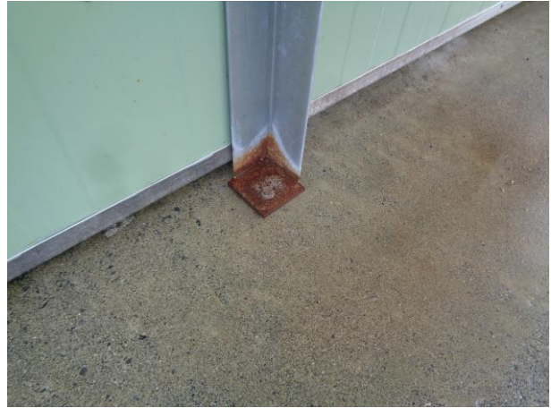
Rust to extract louvre frame support.
