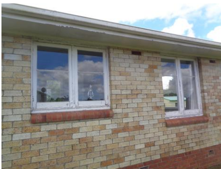
Timber windows poor condition
