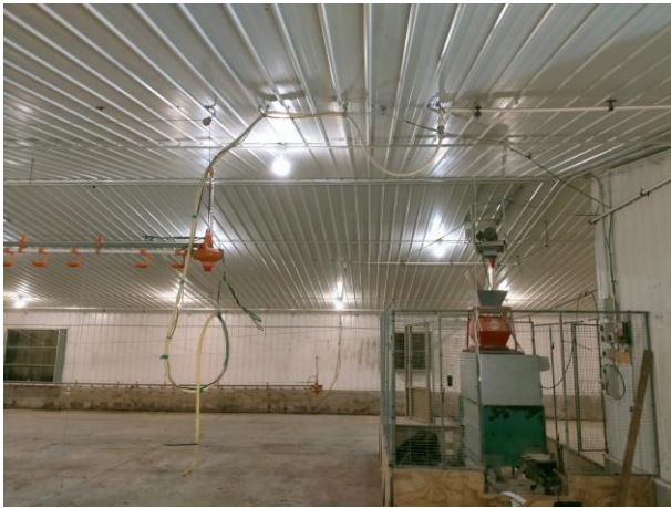
Typical interior construction
