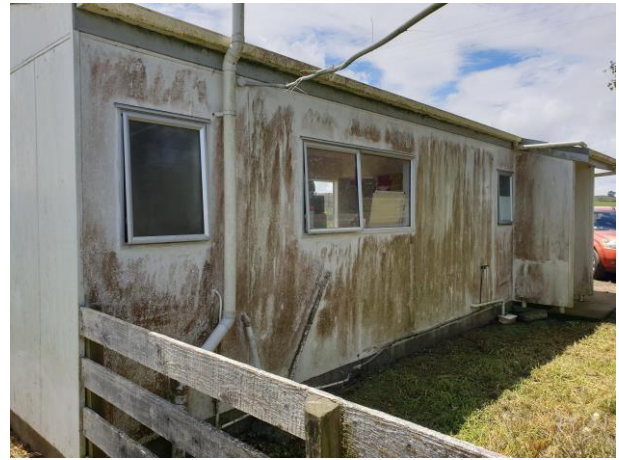
Mould to south side
