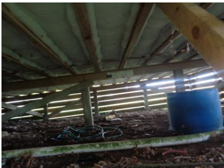
Subfloor insulation. Sheet pvc not required.
