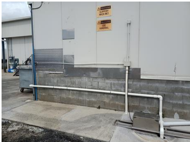
Sheet metal patches to damaged insulated panel
