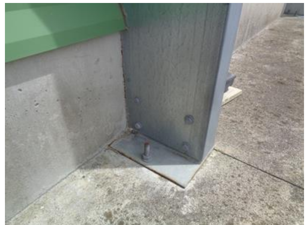
Base plate best on a concrete plinth
