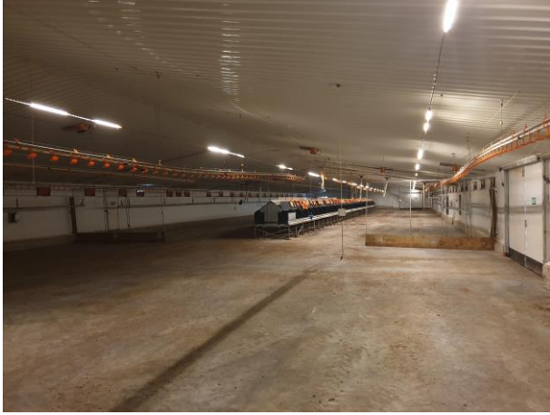
Typical interior view – Shed 7
