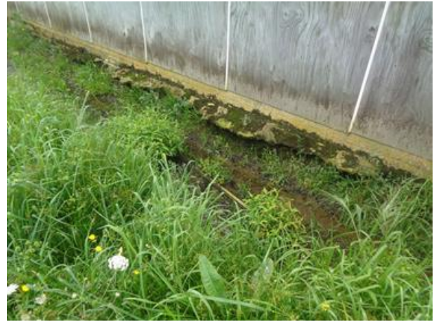
Drainage channel close to undermining slab
