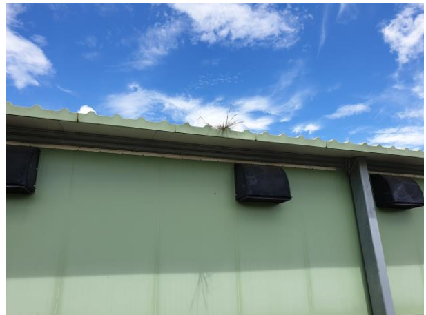
Vegetation growing in the gap between the roofing and the end cap flashing
