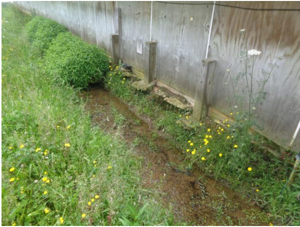
Drainage channel close to undermining slab
