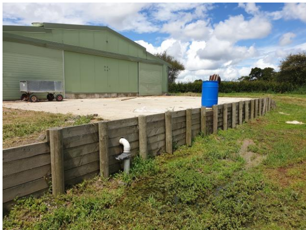
Timber pole retaining wall to rear yard slab showing minor damage to posts and rails
