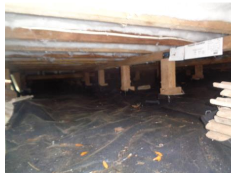
Under floor – insulation and pvc ground cover.
