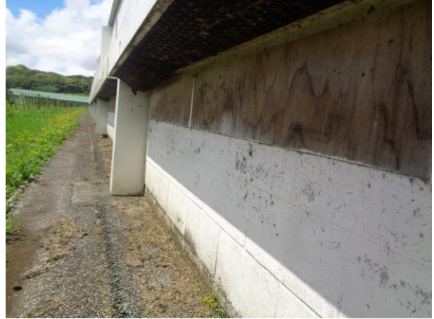
Plywood with no protective coating.
