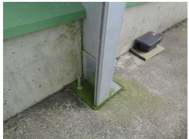
Base plate best on a concrete plinth
