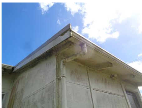
Grime to walls, soffits, downpipes.
