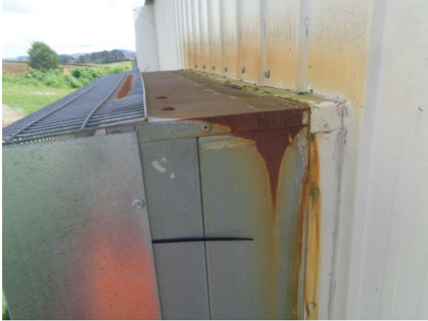
Rusting to top of louvre/fan housing
