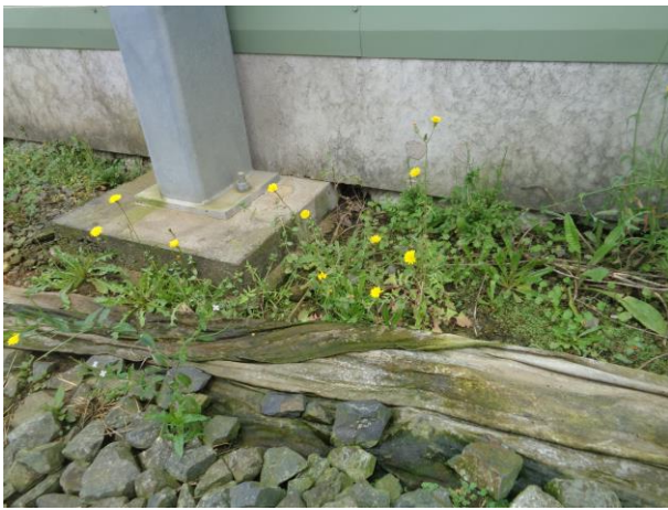
Column base plate best on plinth.
