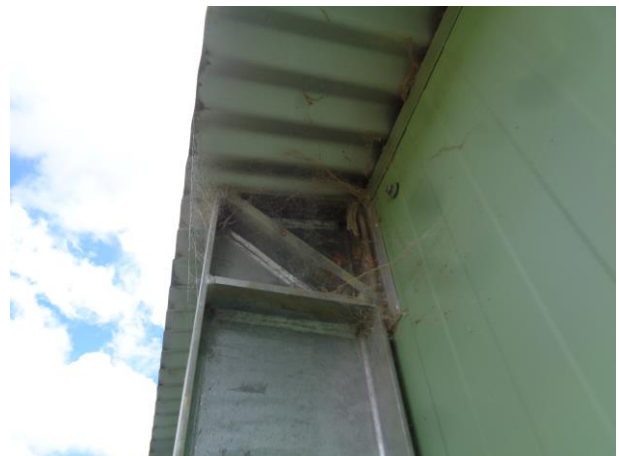
Exterior structural portal leg - galvanized steel
