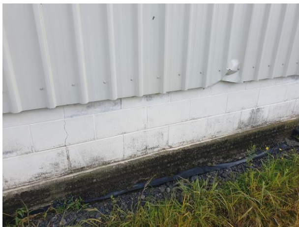
Typical perimeter upstand wall cracking and localised cladding damage
