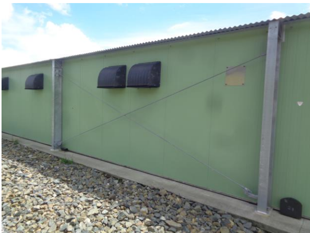
Insulated panel close to concrete slab and not located on a concrete nib.
