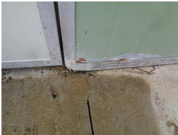
Rust to insulated panel at concrete paving.
