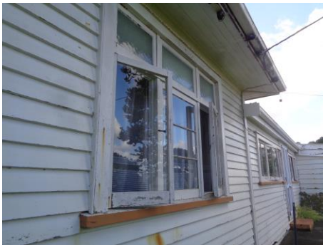
Timber window joinery poor condition
