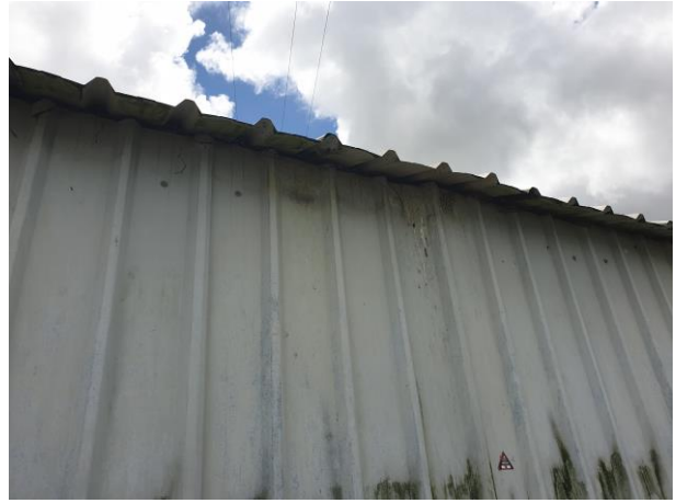
Typical exterior cladding weathering and lack of bird proofing at wall/roof junction
