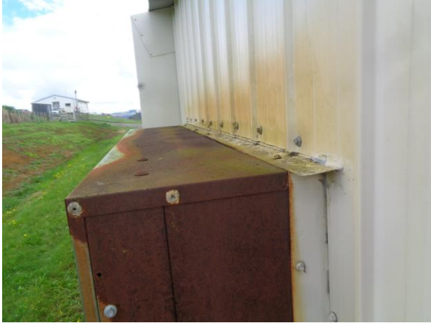
Rusting to top of louvre/fan housing
