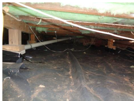
Under floor – insulation and pvc ground cover.
