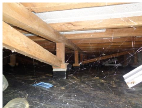
Subfloor insulation and pvc sheet.
