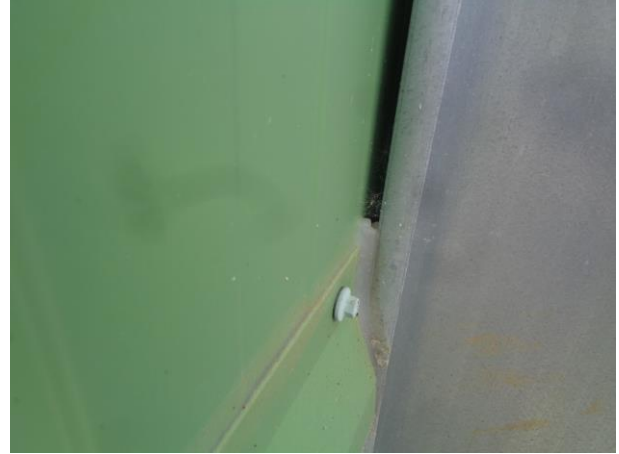
At column gap for water ingress
