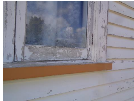
Timber window joinery poor condition
