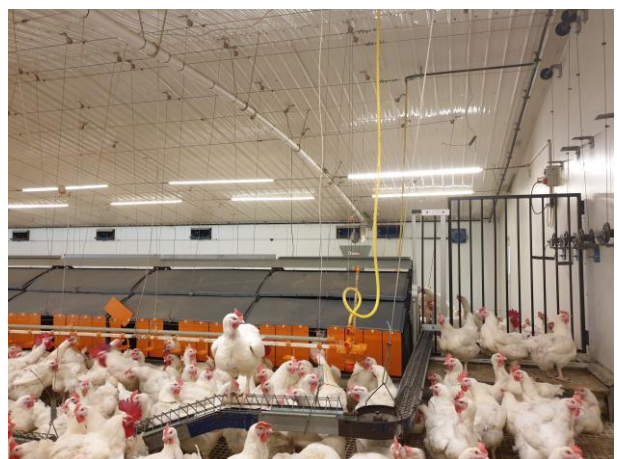
Typical interior construction
