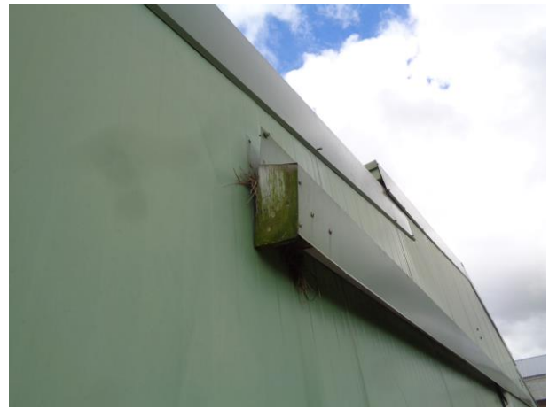
Door track flashing loose.
