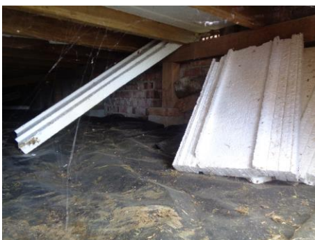
Subfloor insulation dislodged
