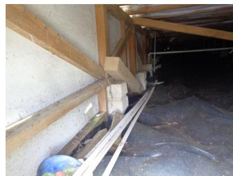
Subfloor space – insulation and pvc sheet. Inside face of subfloor cladding.
