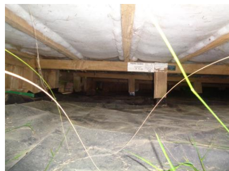
Under floor – insulation and pvc ground cover.
