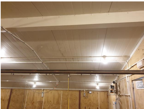
Typical interior construction
