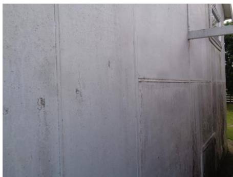
Grime to painted plywood cladding
