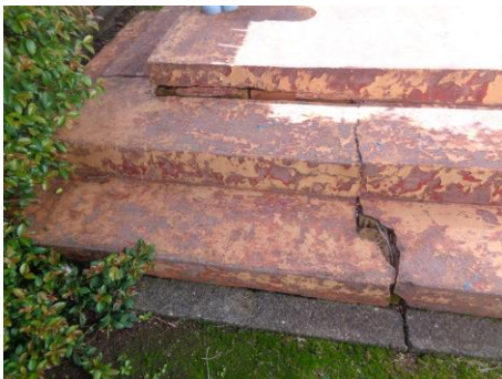
Crack to concrete patio
