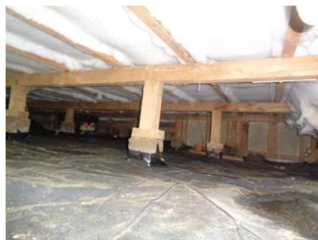
Subfloor insulation and pvc sheet.
