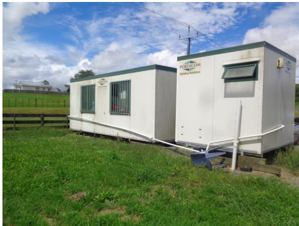
Typical exterior view
