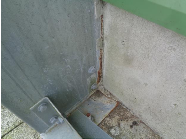
Rust developing at column concrete interface
