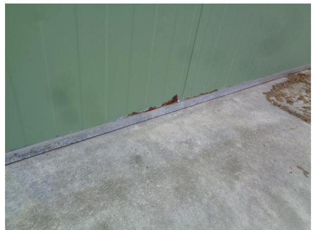
Rust to extract louvre frame
