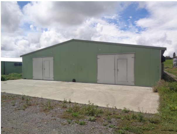
Typical exterior view
