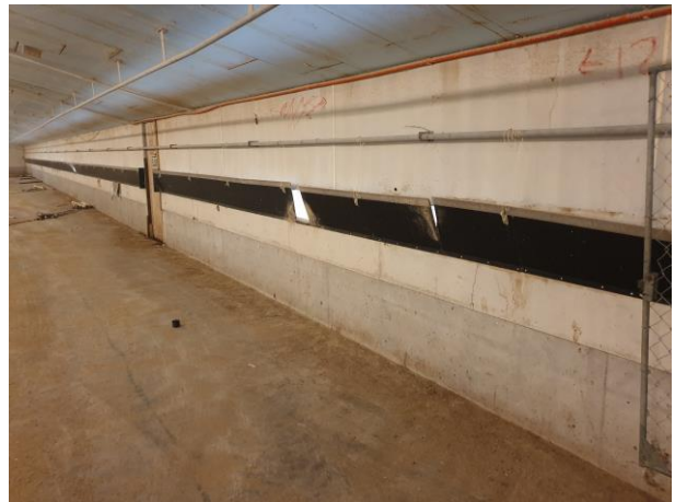
Typical exterior cladding weathering and lack of bird proofing at wall/roof junction
