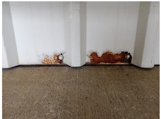
Corroded metal cladding within covered load area. Appears to be timber plate on concrete.
