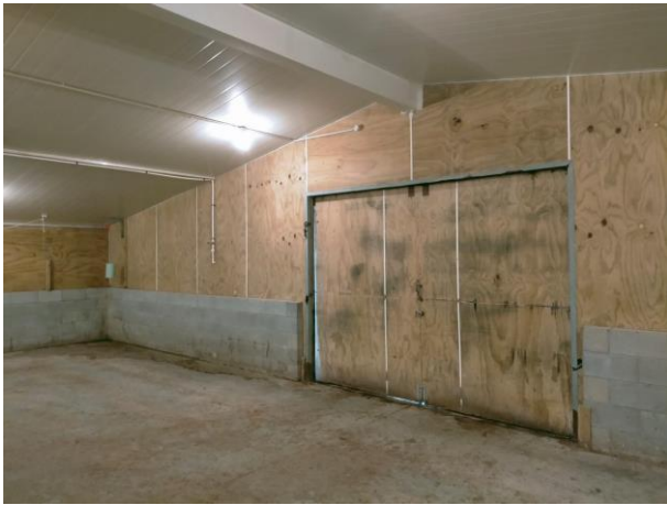
Typical interior construction
