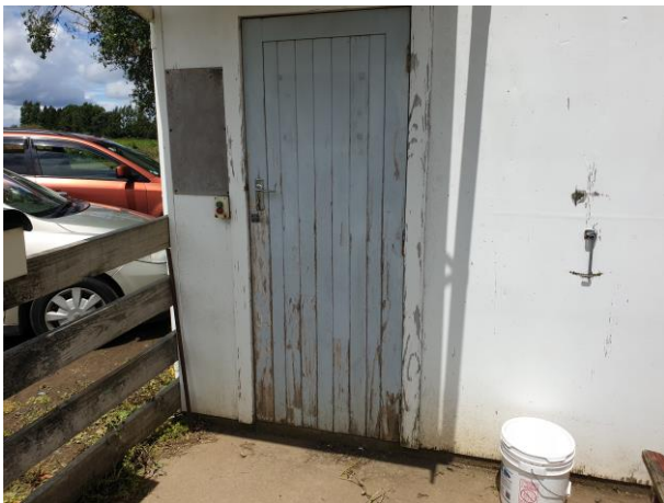
Typical weathering of joinery and cladding
