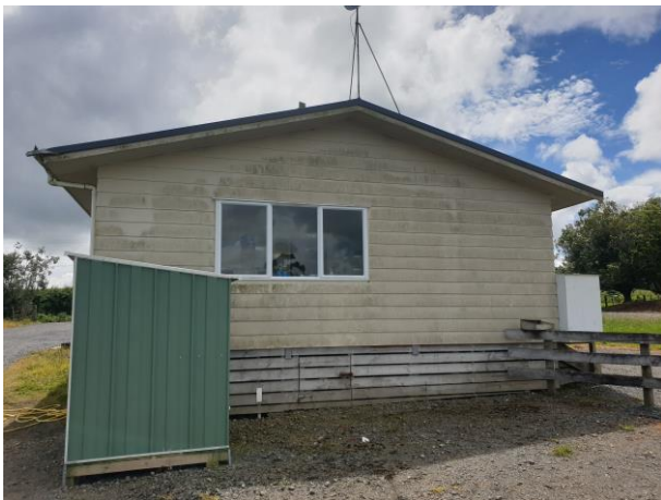
Widespread mould and vegetation in gutters
