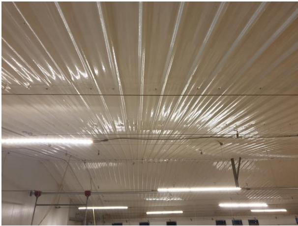
Typical interior construction – Shed 8
