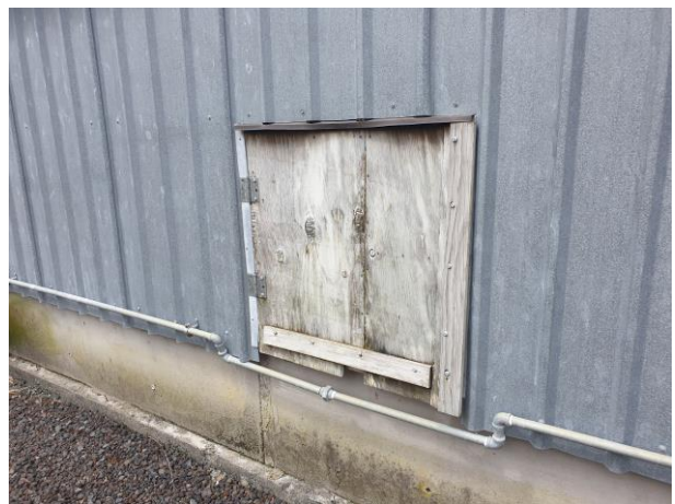
Typical weathering of doors
