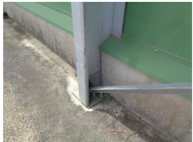
Base plate best on a concrete plinth
