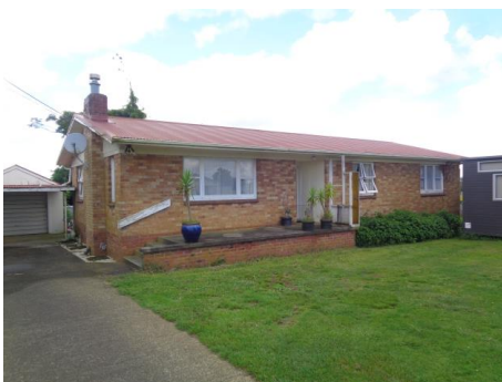
Roof in fair condition
