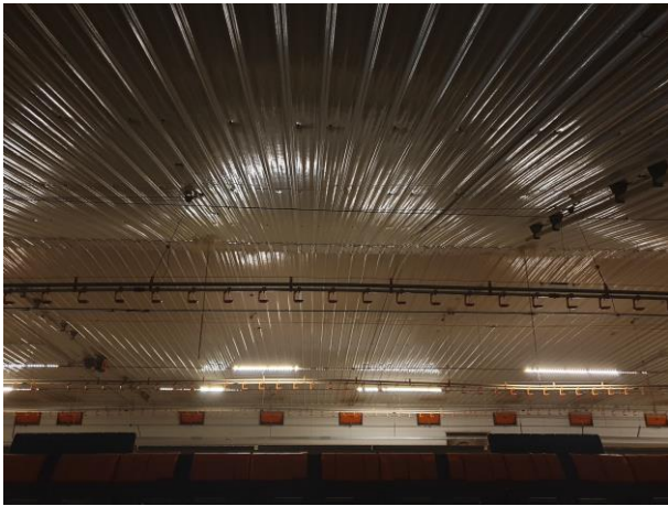
Typical interior construction – Shed 7
