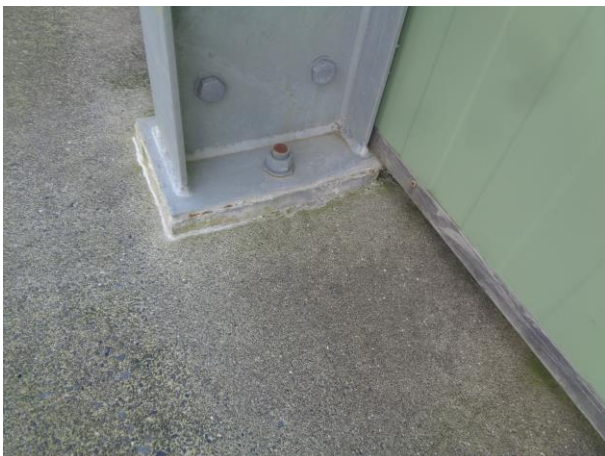
Exterior structural portal leg - galvanized steel
