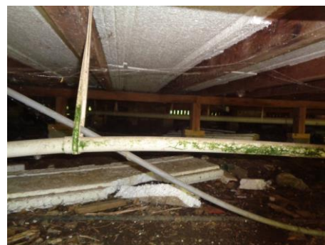
Subfloor space – insulation ( no pvc required)
