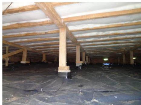
Under floor – insulation and pvc sheet.
