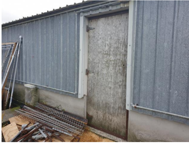
Typical weathering of doors
