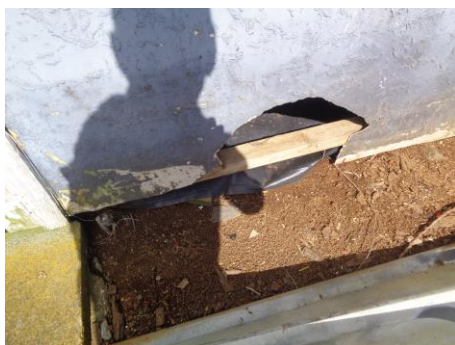
Subfloor cladding damage – possible older James Hardie product containing asbestos.
