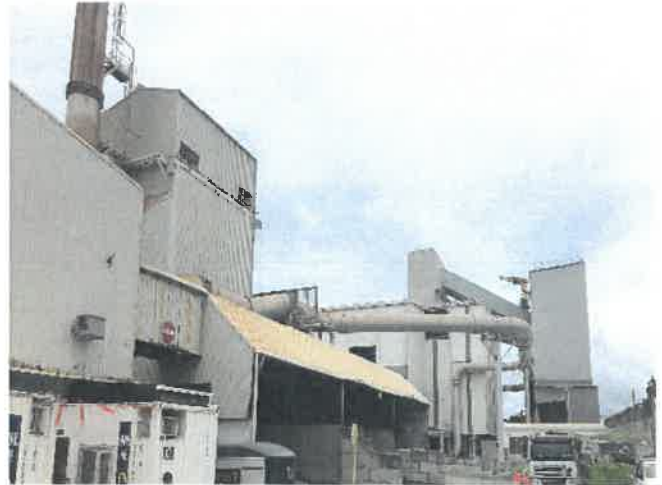
Batch House External – Far Right of picture
