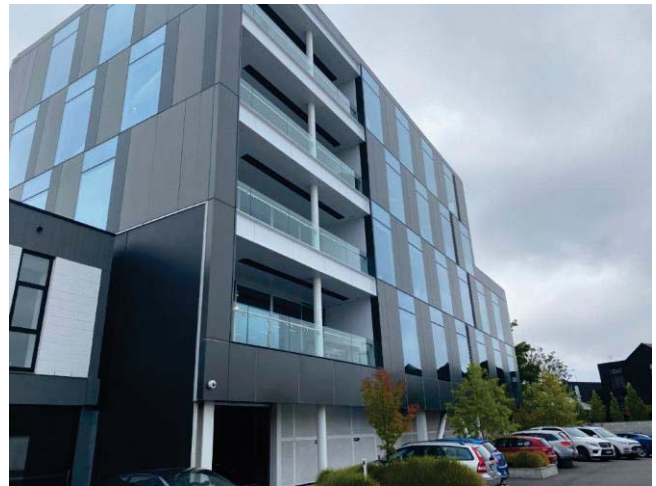
Rear Westwood Lane Façade/Carparking
