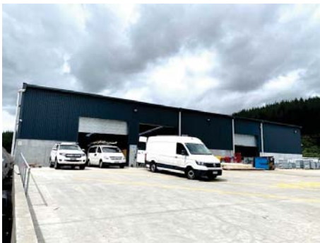
Concrete Ramp to Warehouse
