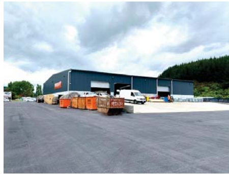
Rear Yard and Warehouse access
